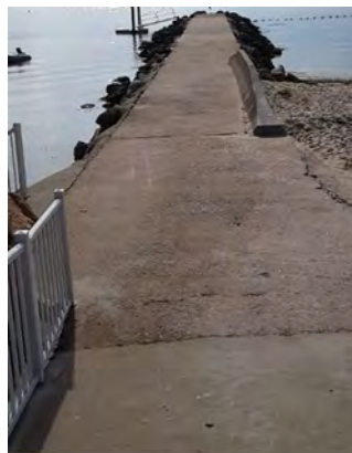
North Groin Paving
