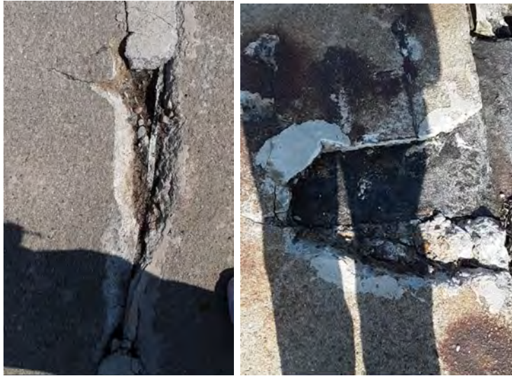
Paving Deterioration
