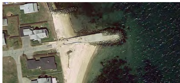
Figure 2 BPtBA - Osprey Pier/Groin
