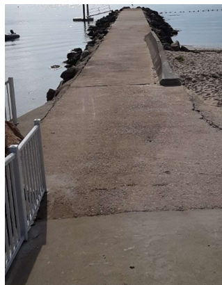
North Groin Paving
