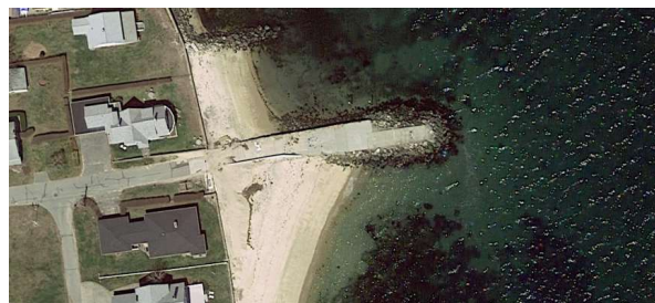
Figure 2 BPtBA - Osprey Pier/Groin
