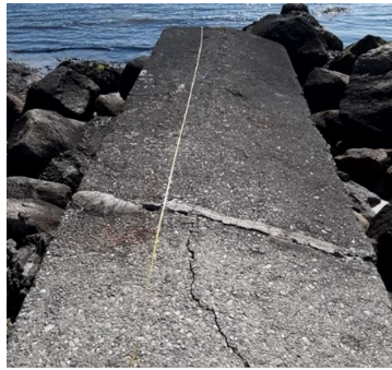
Drainage Pipe Concrete Encasement
