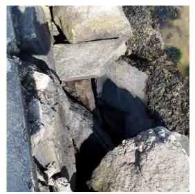
Gap in Armor Stone Revetment Requiring New Stone Infill
