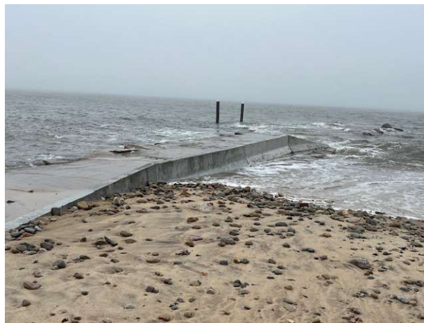
Image 7: South Beach groin, January 2024 (image courtesy of Jan Orsini)
