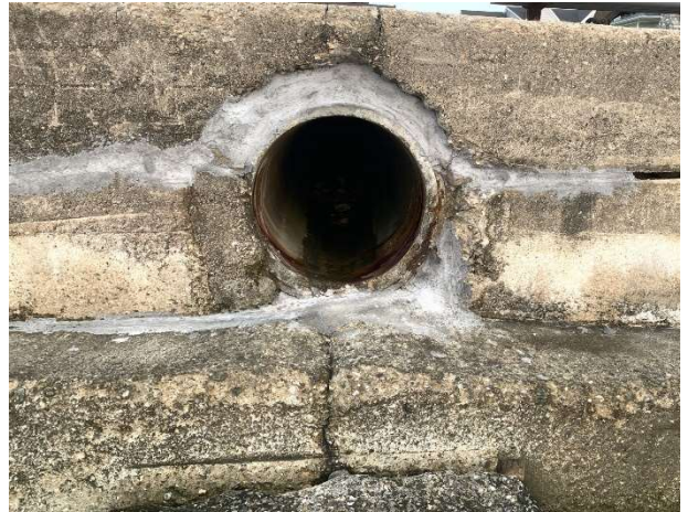
Image 19: Drain outfall (Blue Heron Way, 2023)
